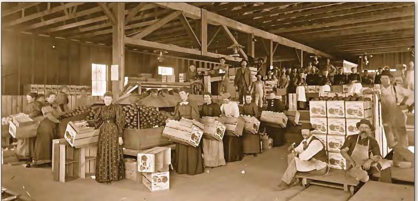
This 1897 scene shows a shed of the Houser Bros. Co. in Covina. They used kerosene lamps for lighting, and the equipment was powered by a treadmill device. The two men in the center standing on top of the sizing machine were the power source.
