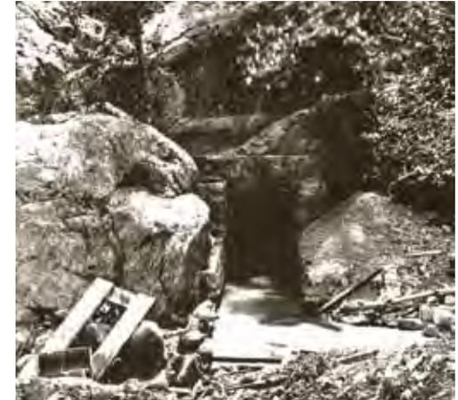
**This photo shows the completion of the work in lining the tunnel with a cement floor to stop seepage.**
