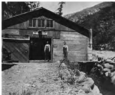
**San Antonio Light and Power plant was built into the side of the canyon wall. This plant made history on Dec. 31, 1892. It was the first commercial application of transformers to effect long-distance, high-voltage transmission of electricity with the use of alternating current.**
