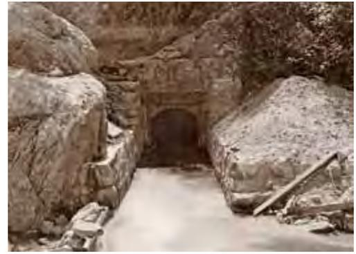
**Water of San Antonio Creek diverted through tunnel and directed into the penstock (high-pressure line to powerhouse).**
