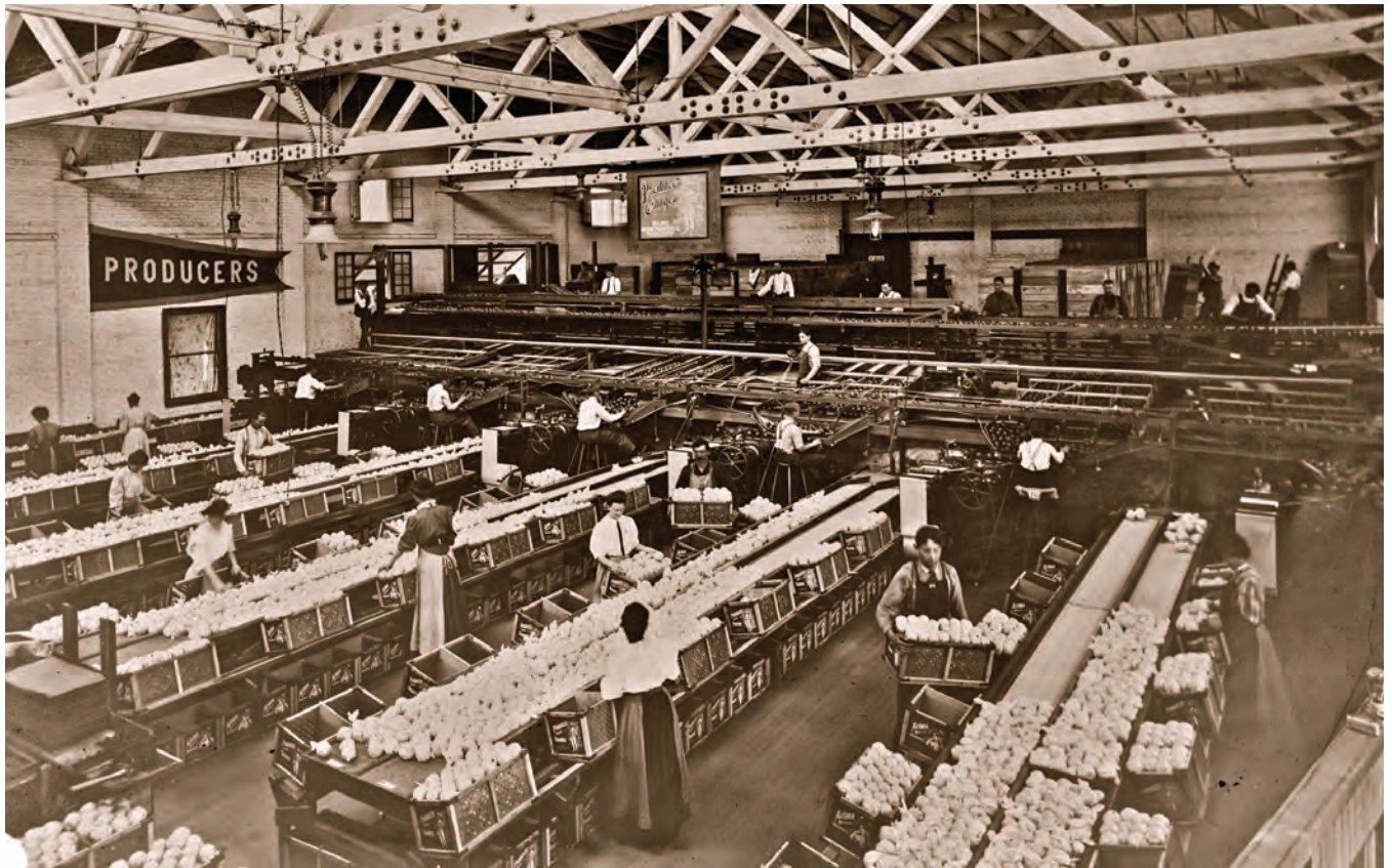
Interior of Redlands Orange Producers packinghouse. They were an early customer of Mill Creek's electricity. (Note arc lighting and electric-powered conveyor belts.)
